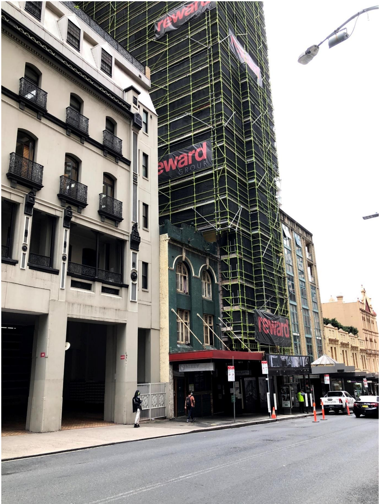
Figure 4: Site viewed from Pitt Street looking south
