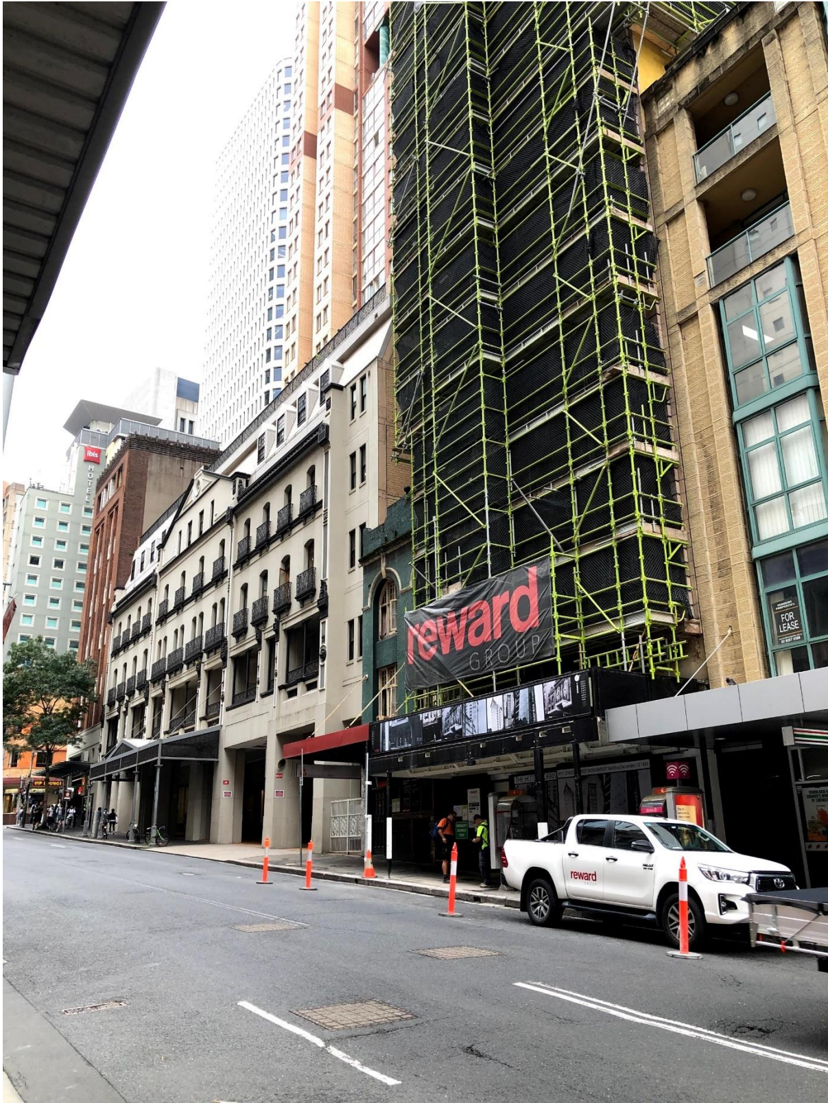
Figure 5: Site viewed from Pitt Street looking north
